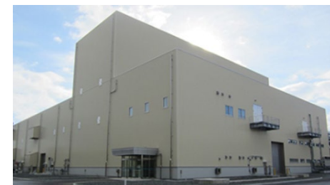
[Japan: Aomori] Vitrification Technology Facility
