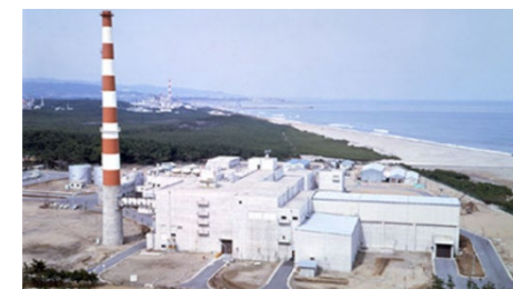
[Japan: Ibaraki] Spent Nuclear Fuel Reprocessing Facility
