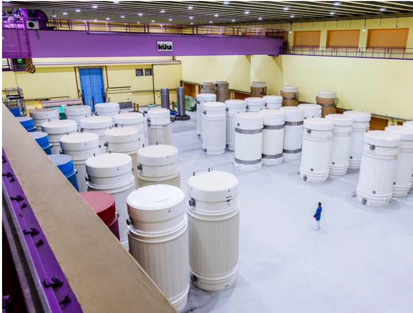
Zwilag Interim SNF Storage Facility, 2800 \text{ m}^2 ( \sim 70 \text{ m} \times 40 \text{ m} ) to store SNFs generated for 50 years from two 1 GW NPPs
